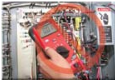
Do not remove or bypass the connections on any electrical circuit.
